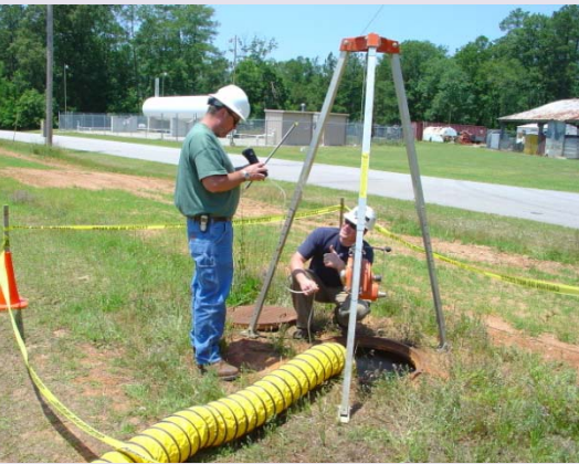
LTI's On-Site Engineers
